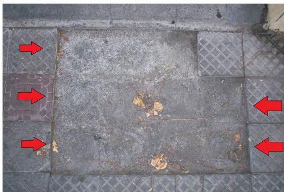
Missing tiles; uneven surface
