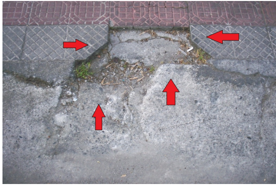
Missing tile; uneven surface
