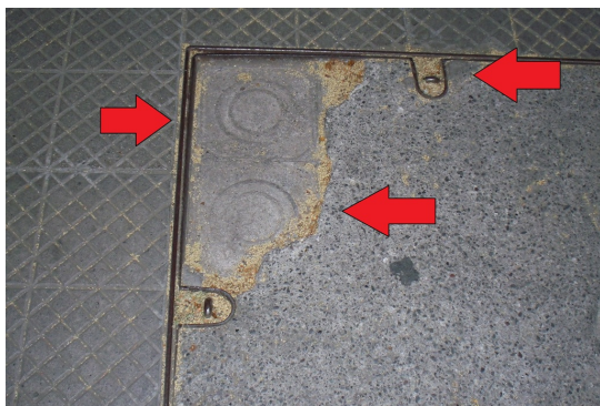
Manhole cover, missing tiles
