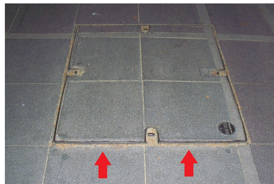
Manhole cover with raised edge
