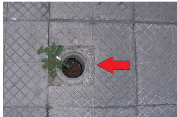
Water meter with no cover; lots of these!
